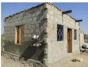
The CONCRETE BRICK shelter is built with reinforced concrete or cement bricks and plastered with cement mortar. The walls need to be at least 8" thick and should be plastered. Care needs to be put in the choice of beams and its placement. Commonly the roof is made of thatch or other structural system, plastic sheeting with a mud plaster layer, protected with a final waterproofing layer.
