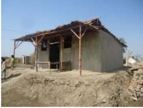
The LOH KAT shelter is built with a supporting skeleton made of timer poles, bamboo or steel. The skeleton is covered with matting and then filled and plastered with mud. Commonly the roof is made of thatch or other structural system, plastic sheeting with a mud plaster layer, protected with a final waterproofing layer.
