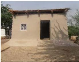
The MUD shelter is built with unreinforced layers of a mixture of mud and straw. The walls need to be at least 18" thick and should be plastered. Care need to be put in the choice of beams and its placement. Commonly the roof is made of thatch or other structural system, plastic sheeting with a mud plaster layer, protected with a final waterproofing layer.
