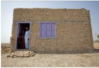
The BURN BRICK shelter is built with fired bricks. The walls need to be at least 9” thick and should be plastered. Care needs to be put in the choice of beams and its placement. Commonly the roof is made of thatch or other structural system, plastic sheeting with a mud plaster layer, protected with a final waterproofing layer.
