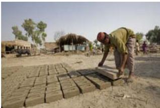
The ADOBE shelter is built with sundried mud bricks. The walls need to be at least 13.5" thick and should be plastered. Care needs to be put in the choice of beams and its placement. Commonly the roof is made of thatch or other structural system, plastic sheeting with a mud plaster layer, protected with a final waterproofing layer.
